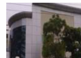
API Facility ANKLESHWAR, GUJARAT
