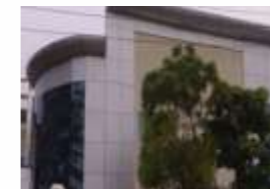
API Facility ANKLESHWAR, GUJARAT
