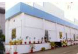
Formulation Facility Unit I KANDLA, GUJARAT
