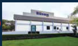
Formulation Facility KANDLA, Unit I GUJARAT
