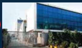
API Facility I ANKLESHWAR, GUJARAT
